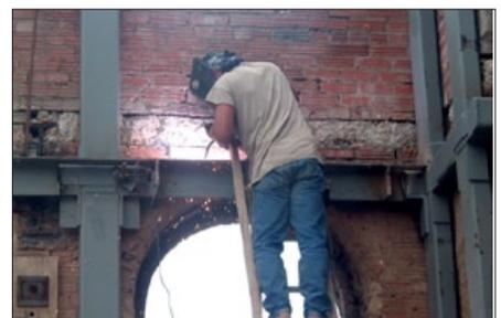
external skeleton to support the existing masonry walls while the guts of the old building were torn out and replaced with a new steel and precast concrete structure.
