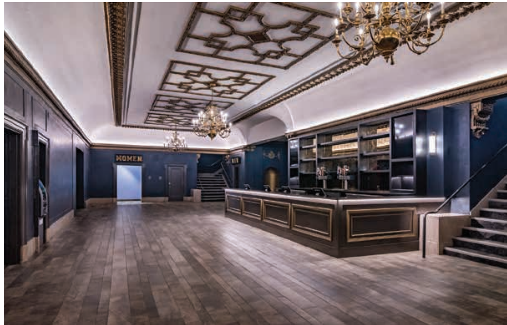
FRESH LOOK In the lobby, gold plaster ceiling details stand out, as do the original rosettes above concrete arches leading up the staircase to the theater balcony. The refreshed space also includes new flooring and a bar with a quartz countertop and custom millwork wood shelving.
