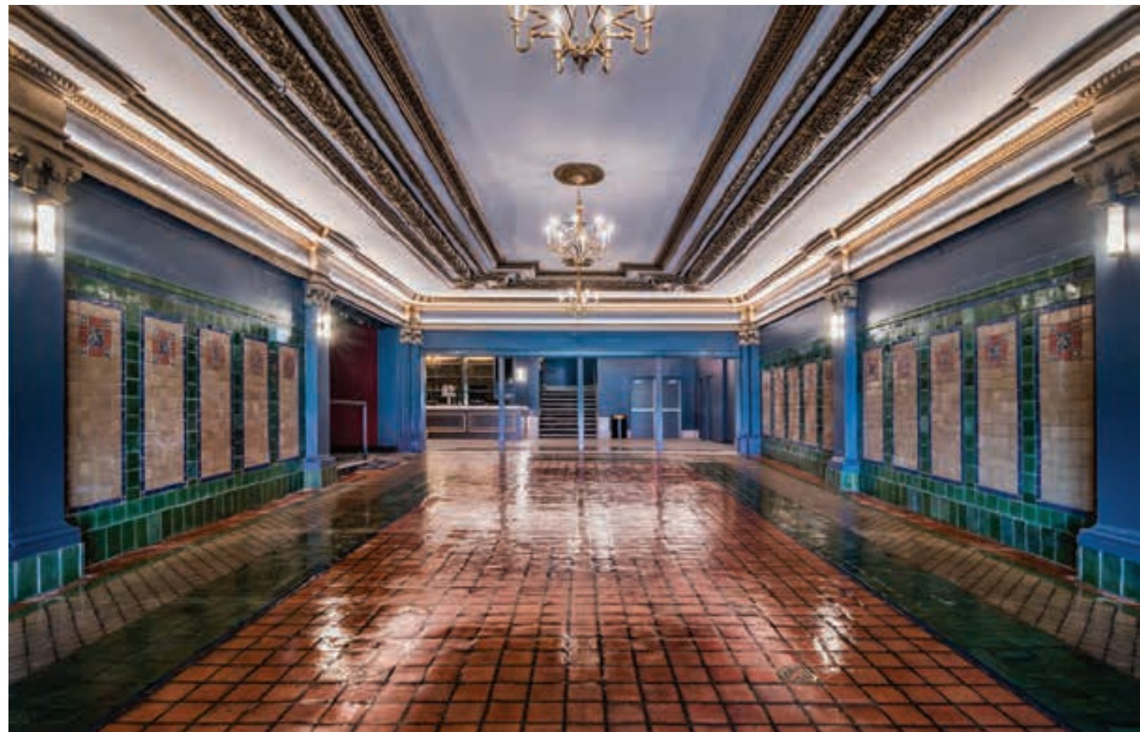
BIG REVEAL During demolition early in the project, workers ripped off black plywood that hid the lobby's original walls and a linoleum-covered wood-framed deck on the floor. They found a sloped floor and walls made of colorful tiles, installed when the building was first constructed in 1913 as the Metropolitan Theatre opera house.
