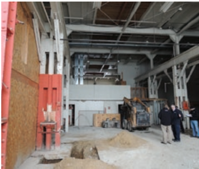
MEASURED APPROACH To assist the construction team (left), a laser scan was performed and utilized to create a three-dimensional digital model from which exact measurements could be obtained at any elevation within the existing structure (right).
